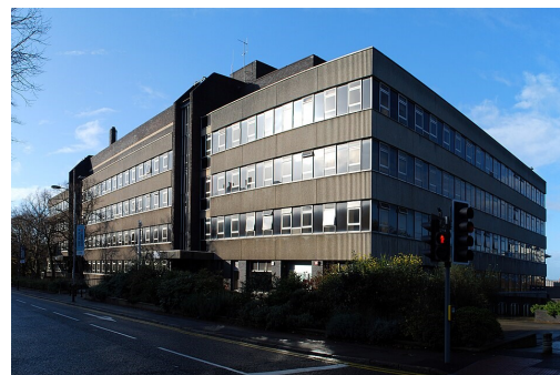
Maurice Shock Medical Sciences Building completed in 1977 on University Road.
